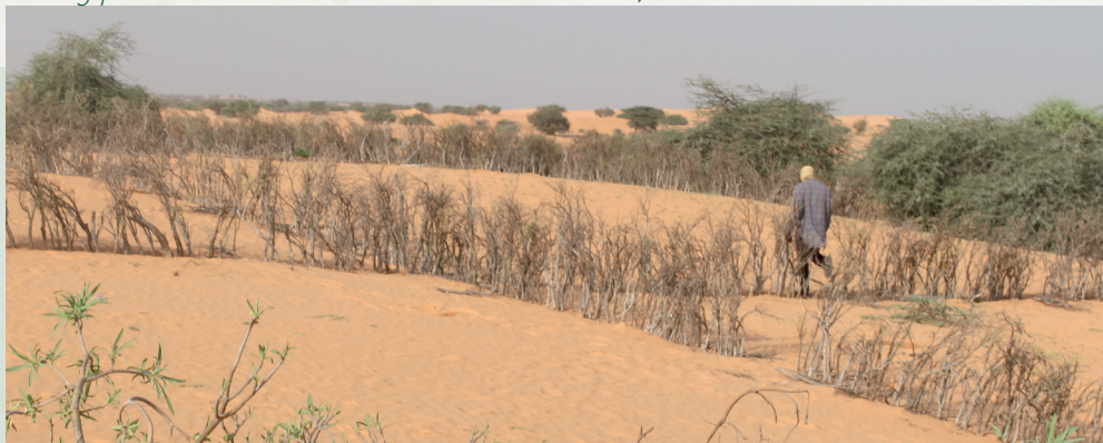
Silting protection installations with native woods, Mauritania
